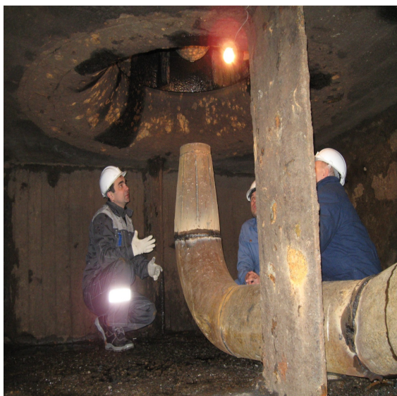
Figure 6. Installation of the annular jet device on the recycling line of the axial pump OPV 2-110 of the Novocherkassk State District Power Station
